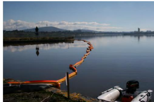
Furlled curtain deployed into water
